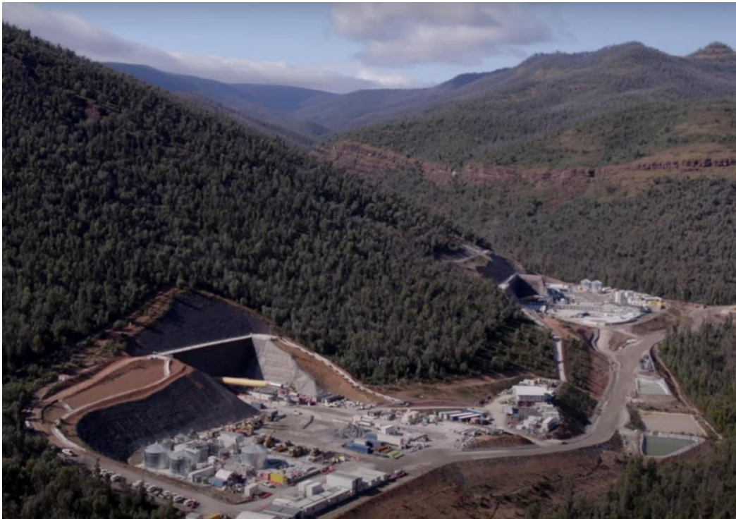
Entrances for two access tunnels to underground station
