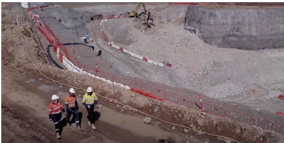
Works at Tantangara Reservoir
